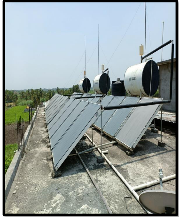
Solar Water Heater Facility
